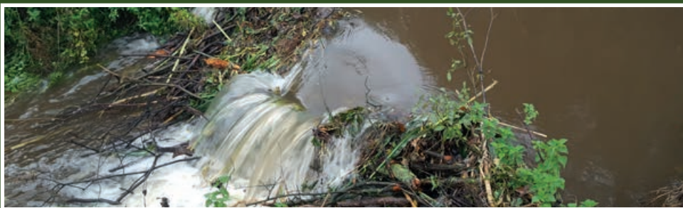
Impounded water caused silt to be deposited in a drinking bay that had been constructed to restrict cattle access to the river.
