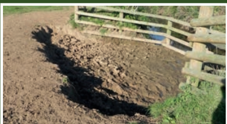
Impounded water caused silt to be deposited in a drinking bay that had been constructed to restrict cattle access to the river.
